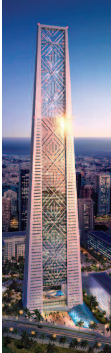
Artist's impression of the 400 metre, 66-floor Lighthouse Tower approved for construction in Dubai, United Arab Emirates. Designed by the Welsh School of Architecture and partners within the new Welsh Low Carbon Research Institute, it aims to achieve a major reduction in energy use compared with a standard high-rise building. There will be three large 225 kW wind turbines, 29 meters in diameter, on the building's south facing side to generate electricity. It will also be clad in 4,000 solar panels to generate additional electricity. The tower will also reduce its overall energy consumption by 65 per cent, and its water consumption by 40 per cent in comparison with an equivalent building.
