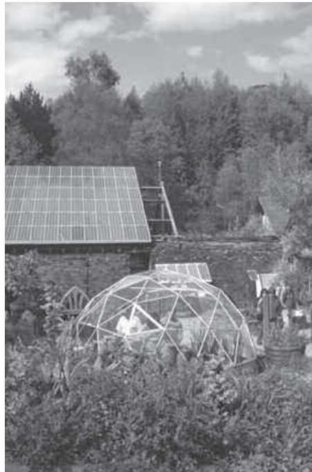
There is considerable potential for micro-energy systems such as the solar panels seen here at the Machynlleth Alternative Technology Centre.
