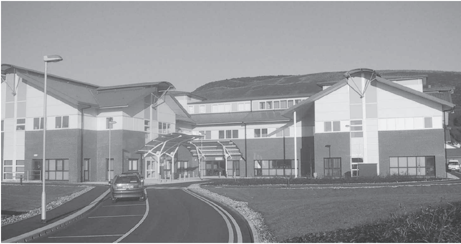
Open in December 2002, the new 70-bed, £66m Neath/Port Talbot Hospital at Baglan was built under a PFI Scheme by Baglan Moor Health Care Limited for Bro Morgannwg Health Trust. Complete with a 24 hour accident and emergency service, it will revert to public ownership after 30 years and repayments totalling £275m.
