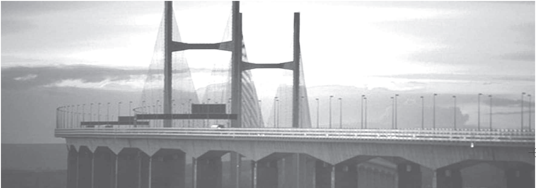
The Second Severn Crossing – in future such major capital projects will be unlikely to proceed without PFI.
