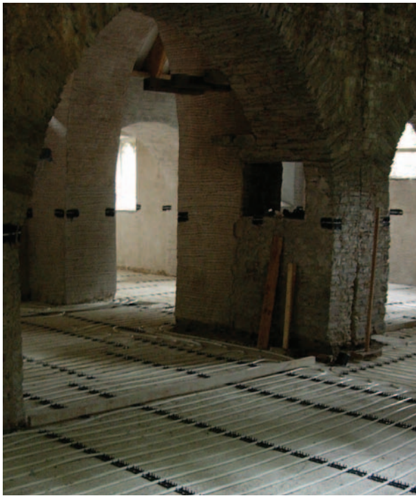
The floor of St Teilo's showing a layer of geotextile as part of the insulation.
