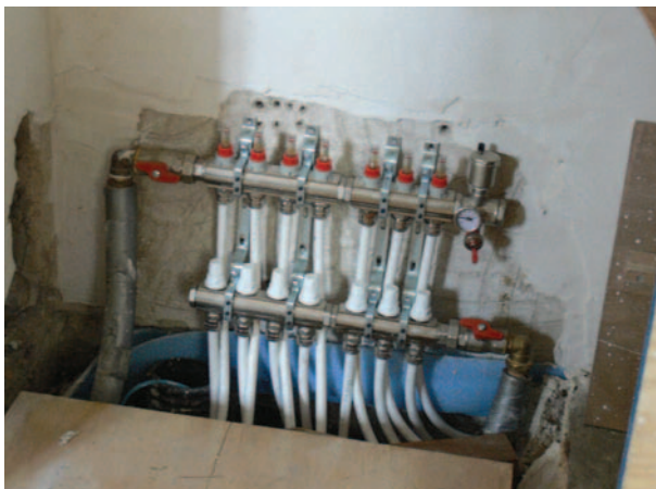
Some of the interior pipes, part of the heating system.
