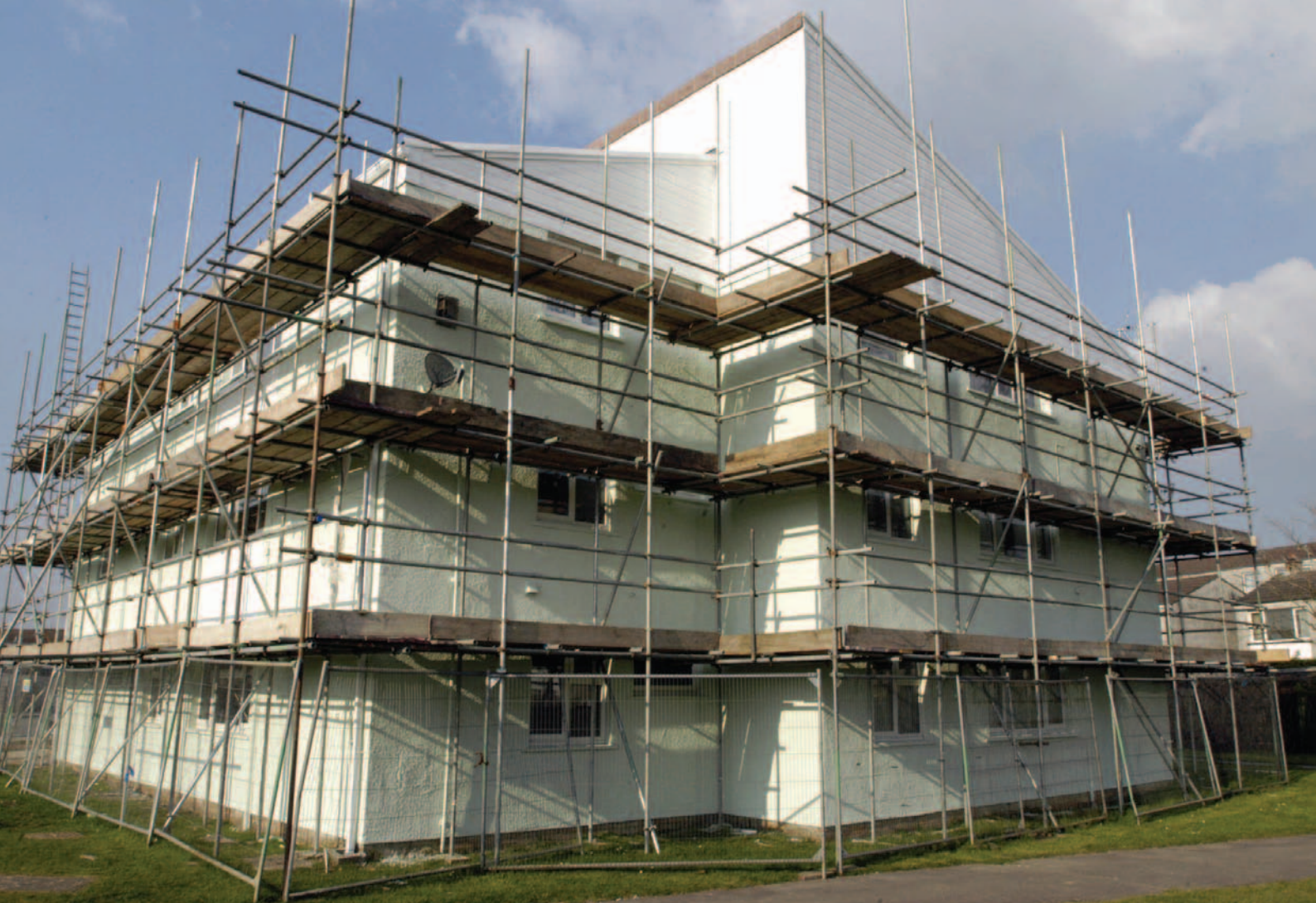
Renovation underway by the Valleys to Coast Housing Association in Bridgend where satisfaction levels among tenants with improvement works is running at 90 per cent.
