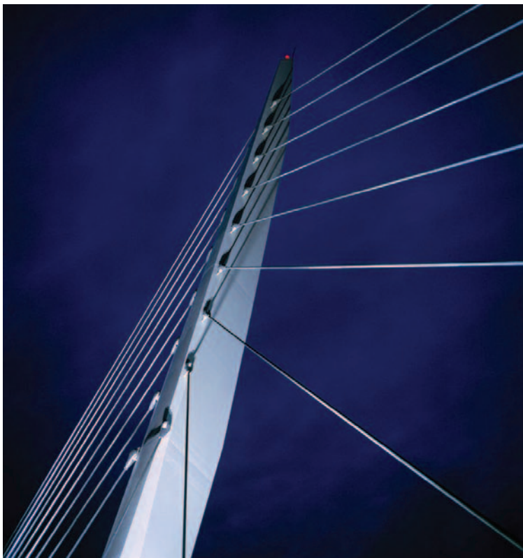
Close-up of the iconic footbridge across the Usk at Newport, creation of the Rowecord company.
