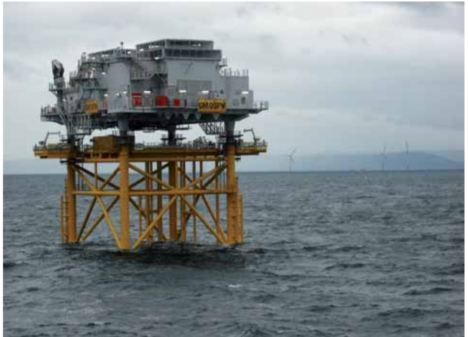
One of the two offshore substations at Gwynt y Môr in Liverpool Bay.
