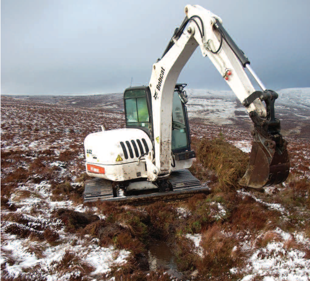
Filling in drains at the Lake Vyrnwy nature reserve in the Berwyn Mountains.
