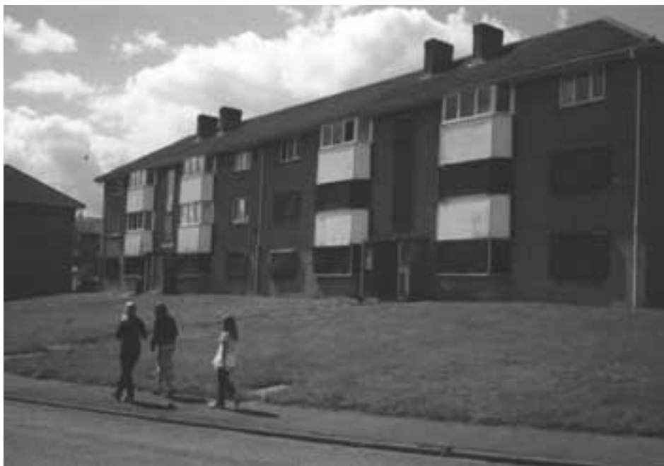
A number of the abandoned houses in Gellideg.
